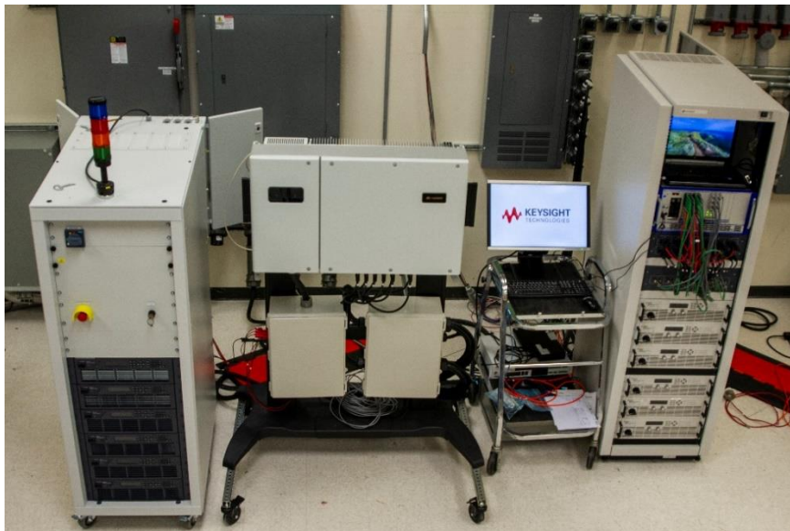
Figure 8. SL1202A AC Emulator with PV8900A Solar Array Simulators and DG9000A PV software.
